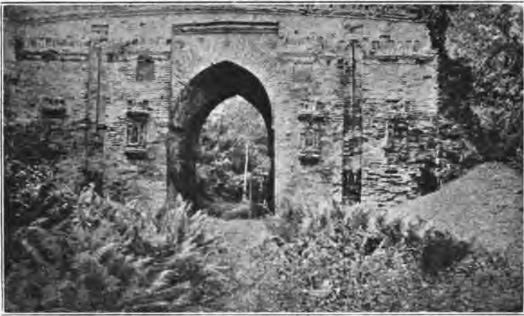
LAST REMAINING GATEWAY TO THE OLD KACHĀRI FORT AT DIMĀPUR.
