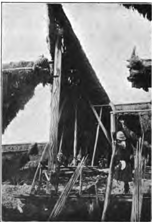
THE MORANG AT NOKCHING, WESTERN PATKOI, WITH HUGE CARVED SERPENT ON FRONT SUPPORTING TIMBER 35 FEET HIGH.
